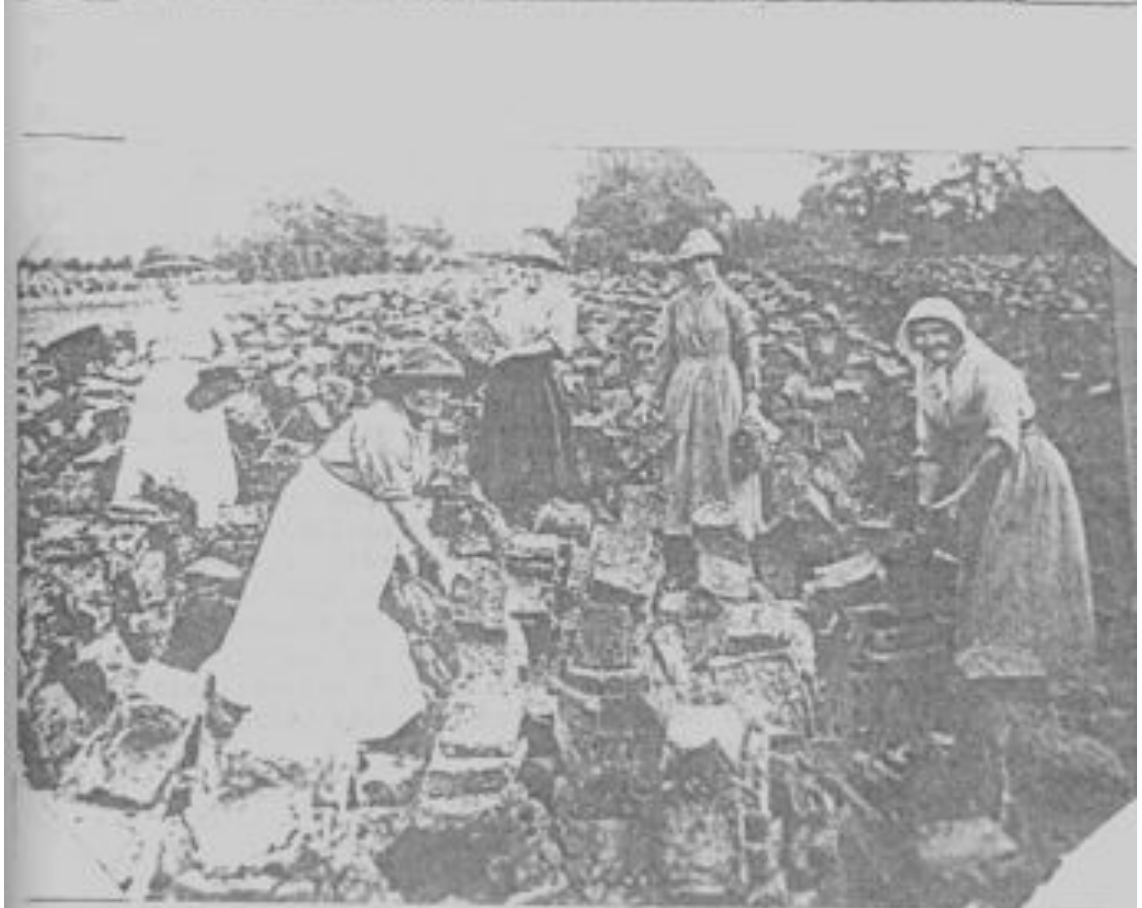
(1) Turf cutters at work, one cutting and the other spreading the cut turf.
