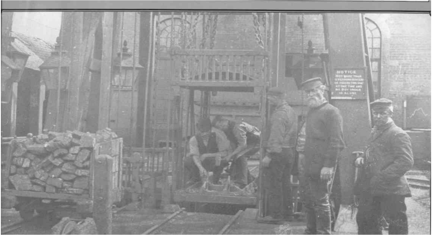
Workmen repairing a cage at Linby Colliery, Nottinghamshire, c.1895. Note the small safety gates about 2ft high and the ornate gas lanterns for lighting. The bearded men are probably officials and the clean-shaven men were ordinary workers. The capes worn were fashionable in the 1890s.
